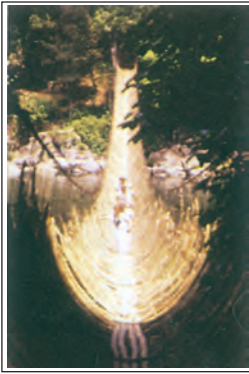
Figure 6.7 : Rope Bridge (Arunachal Pradesh)
